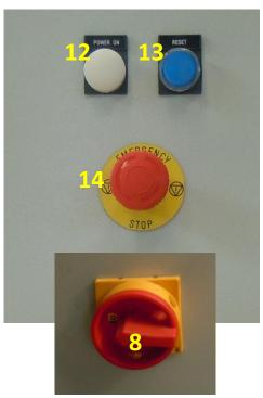
Figure 8 Control Panel Exterior
